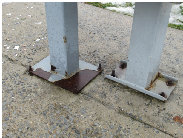
Mailbox station rust and finish deterioration
