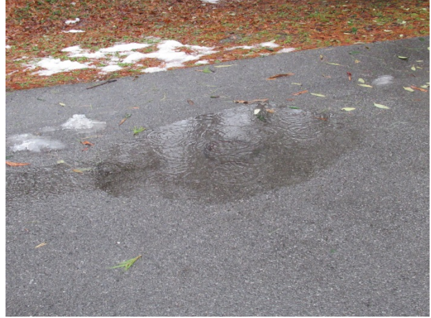
Pavement settlement and ponding water at Ambler Lane North
