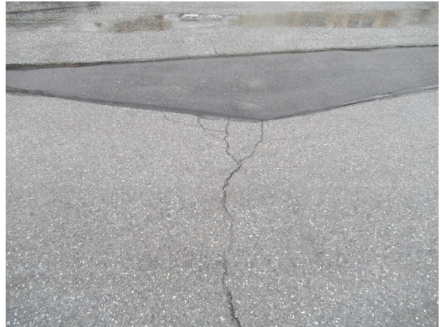
Cracks and patching at Morningside Drive
