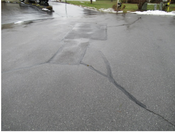
Patching and crack repairs at Whippoorwill Lane
