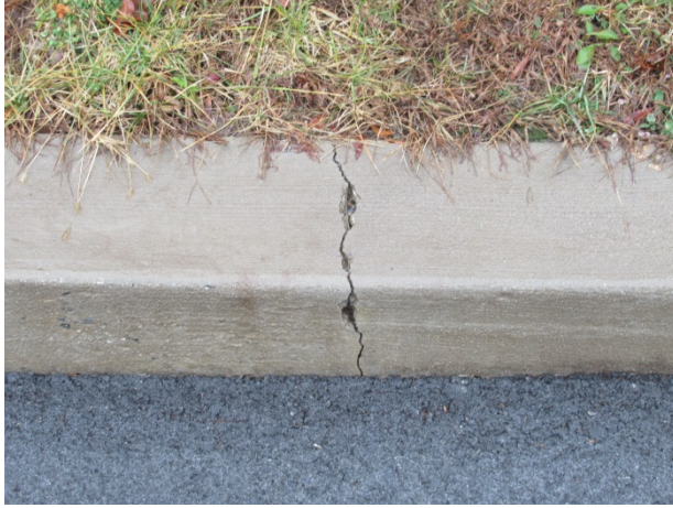
Concrete curb crack
