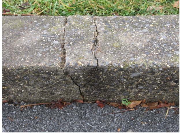
Concrete curb cracks
