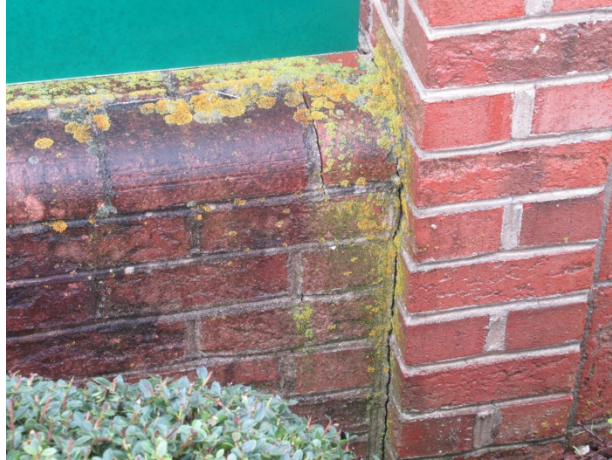
Masonry organic growth and cracks
