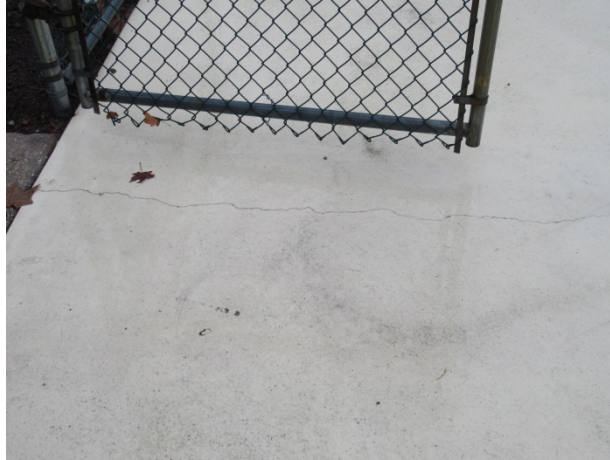
Deck crack
